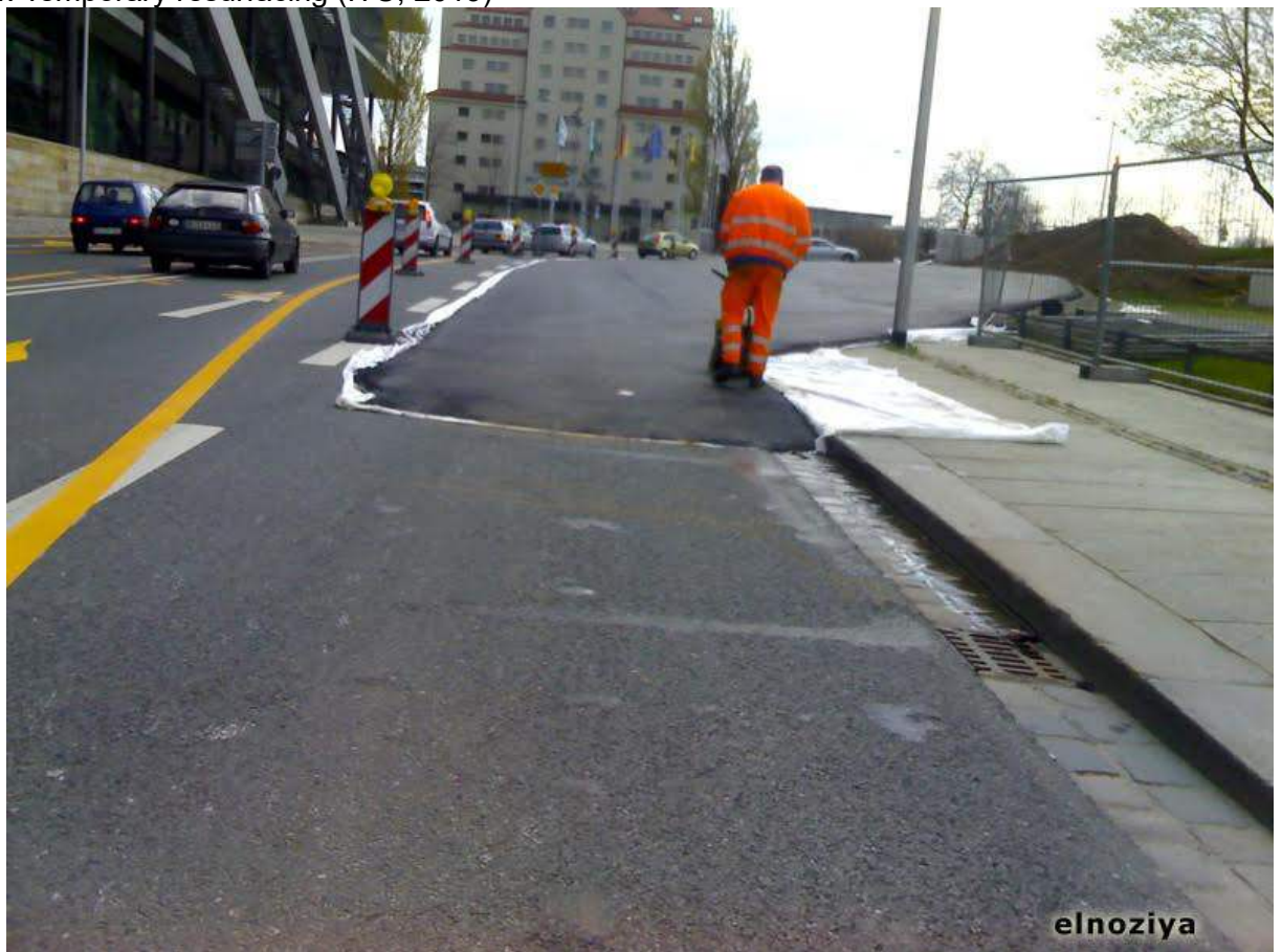
Picture 54: Temporary resurfacing (ITU, 2019)
